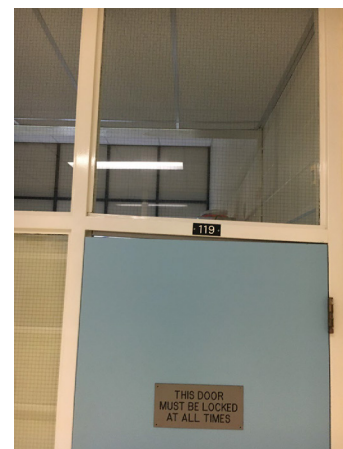
Photo 4: Door frame distorted due to slab heaving
