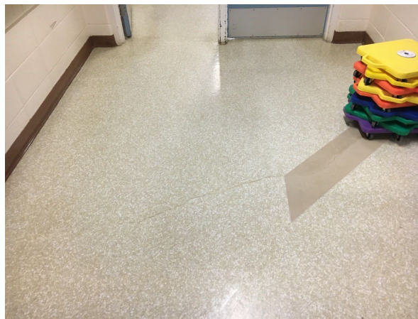
Photo 3: Slab cracking telegraphing through hallway vinyl floor covering
