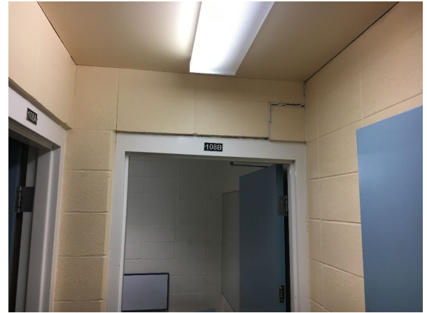
Photo 6: Masonry cracking of header above Room 108B door frame
