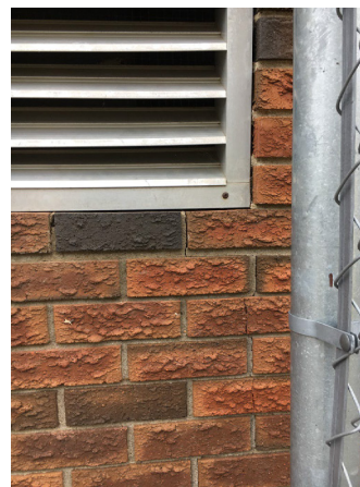
Photo 7: Cracking of brick veneer at mechanical room louver opening
