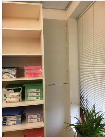
Photo 1: Vertical and horizontal cracking of interior wall at intersection with exterior wall (Room 117)
