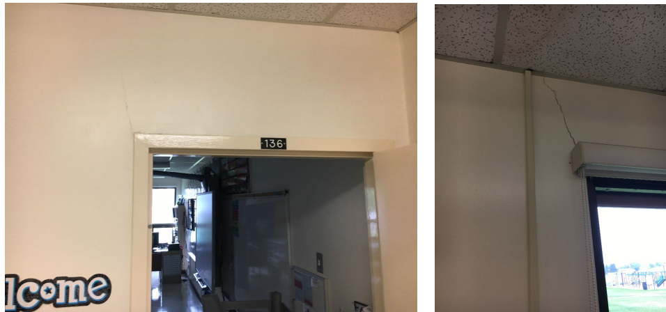
Photos 8 and 9: Minor drywall finish cracking over door and window
