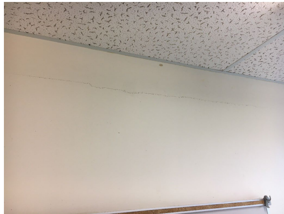
Photo 10: Horizontal finish crack above whiteboard in Room 138
