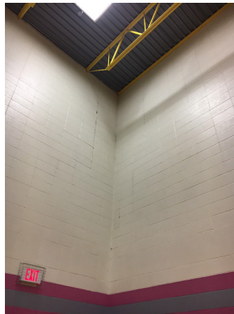
Photo 5: Vertical masonry cracking at corners of gym walls
